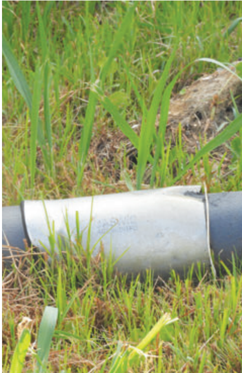
Incorrect use of a stainless joint casket clamp at Elandsrivier cul de sac has led to vast amounts of drinking water being wasted.
